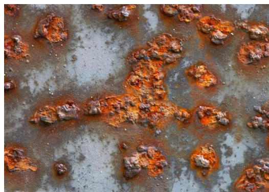
Figure 0.6: Image showing intergranular corrosion ( https://steelfabservices.com.au/intergranular-corrosion/ )
