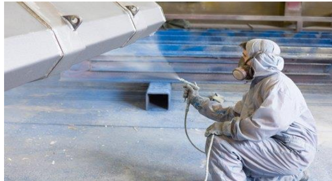
Figure 0.10: Blasting and painting used as a corrosion control measure ( https://www.dookwuise.com/corrosion_control.php# )
