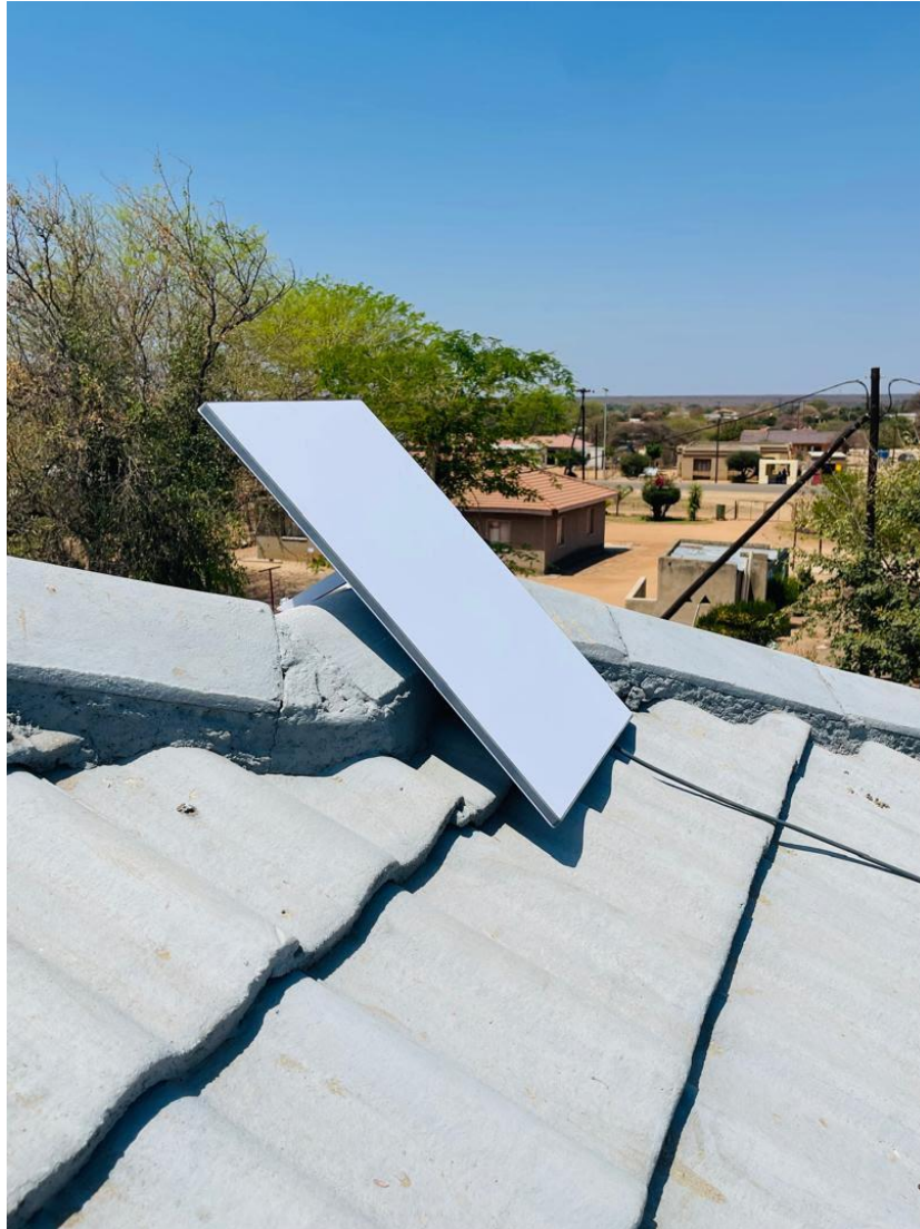
Figure 2. Starlink installtion in Malolwane, Kgatleng District. (courtesy Malakana Interprises).
