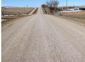
Figure 2: Example of a very good gravel road [1].
