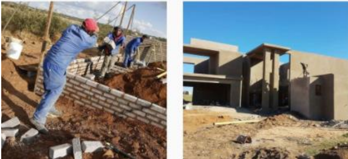
Figure 6 Building construction in Botswana
