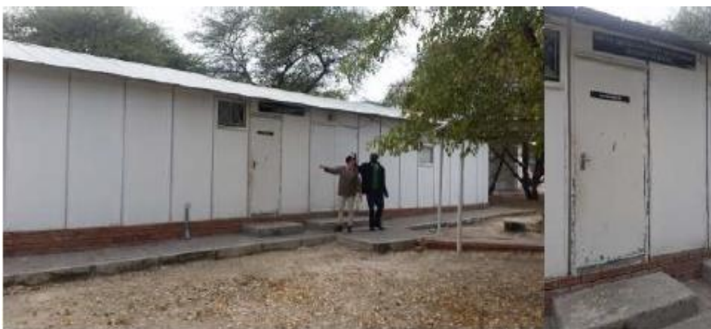
Figure 10 Current Herbarium prefabricated building structure (left) and herbarium entrance (right)
