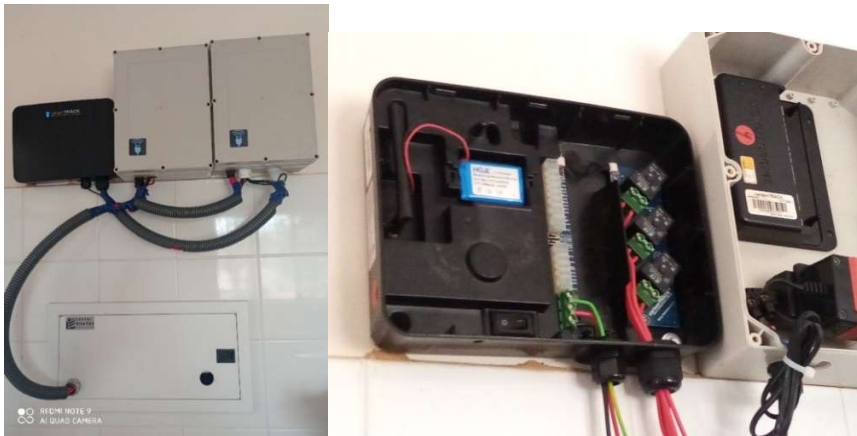
Figure 3.3: The installation schematic of the energy measuring equipment in the house in the experiment.
