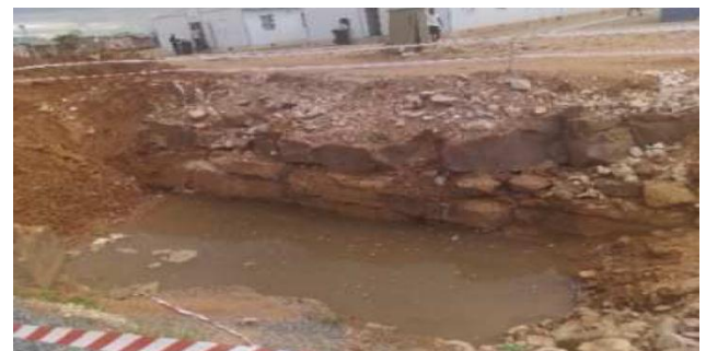
Figure 1: Flooded trench in BIUST
